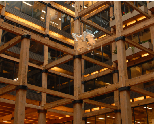
Butler Square | Photography: Preservation Alliance of Minnesota
